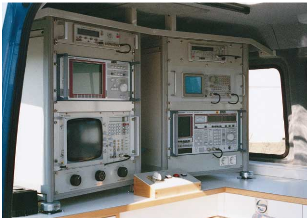
FIG 2 The van contains all equipment required for functional checks on transmitter installations, much of it from Rohde & Schwarz. Photos: author
